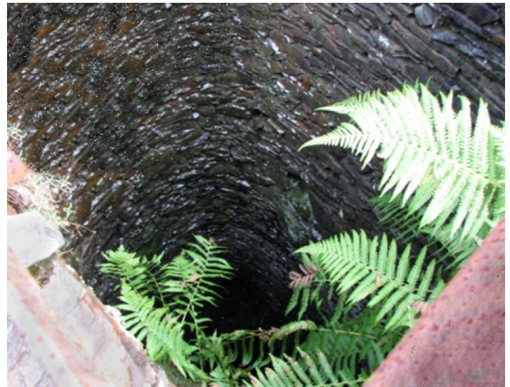
Figure 629: Logaulas mine site. (left) Remains of opencast workings and a shaft. (right) A very well constructed shaft on the hillside to the south of the opencast workings. This shaft was probably equipped with ladders and provided access for the miners.
