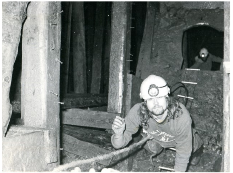
Figure 624: (left) Entrance to Lefel Fawr. (right) Near-vertical shaft connecting Level Fawr to the Kingside level at the location marked '*' in fig. 623 above. To the left is the railway track for raising skips of ore. To the right are a series of timber platforms for the ladderway used by miners.
