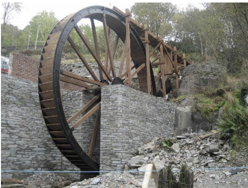
Figure 628: Pontrhydygroes. (left) Water wheel powered by the outlet stream from the Lefel Fawr. (right) Lefel Fawr adit.
